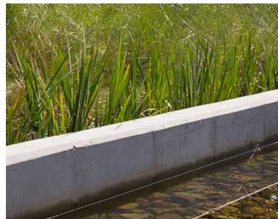
concrete site walls
